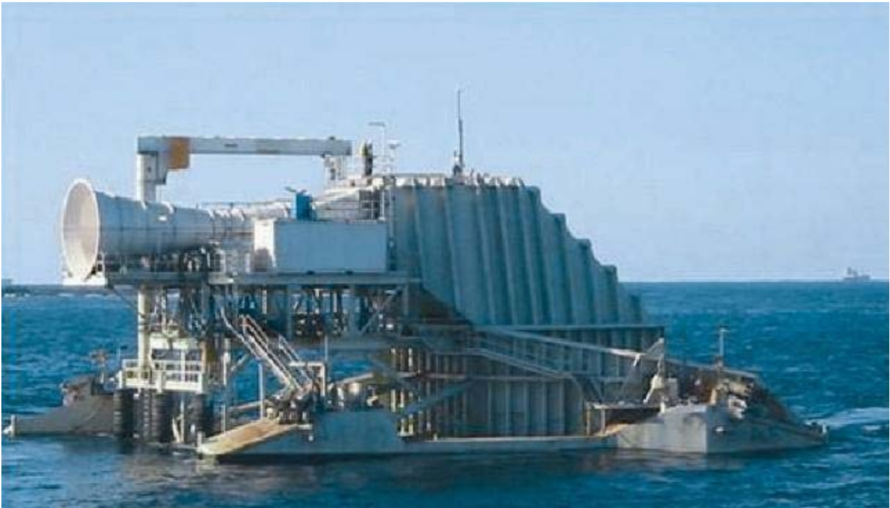
Oceanlinx Wave Power Plant (Australia)
